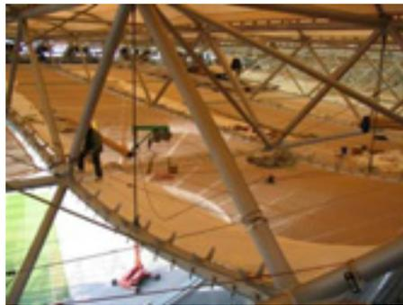
Fig.18. The lower membrane. (View inside the roof box)
