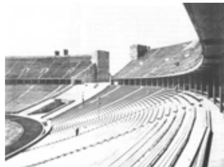
The upper and the lower terraces are structurally completely independent from each other. In tangential direction dilatation joints were provided every 3 or 4 radial frames (i.e. at a distance of 15 to 20 m); they were realised by using brackets. Most of the damages that occurred within the reinforced concrete construction during the 65 years were located at these joints.
