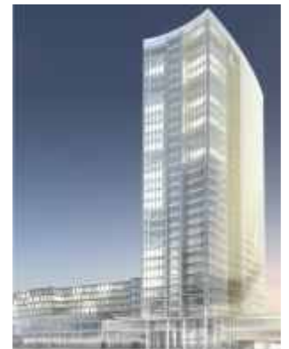
View of office tower
