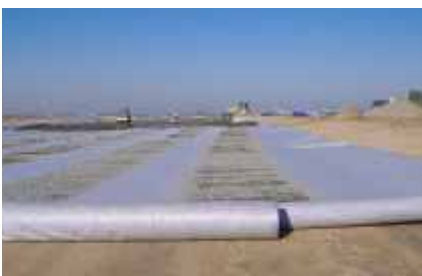
Laying of fleece on Apron 4
