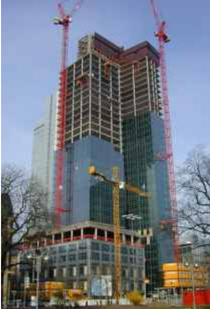
Shortly before completion of the last slab
