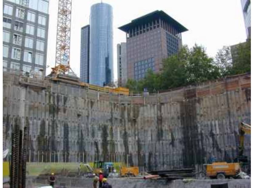
Walls of the construction pit
